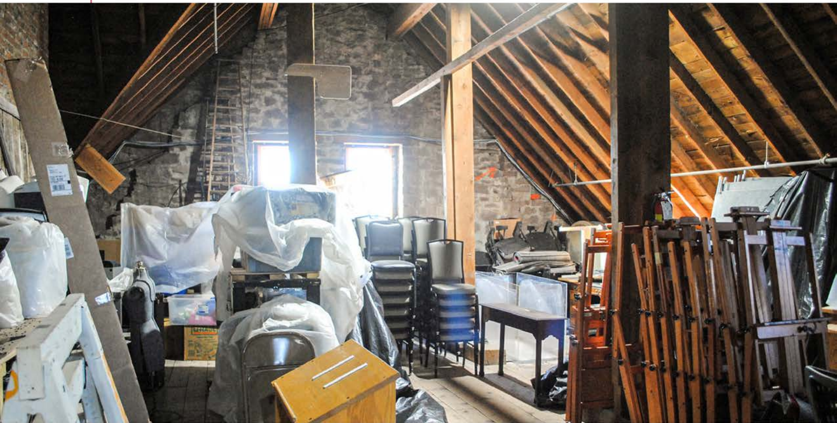
Southwest corner of the historic attic, taken December 2022.
